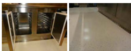
An undercounter fridge unit built into a mega-yacht galley, in accordance to US PHS standards (above left) Resin floors are ideal for mega-yacht galleys (above right)
